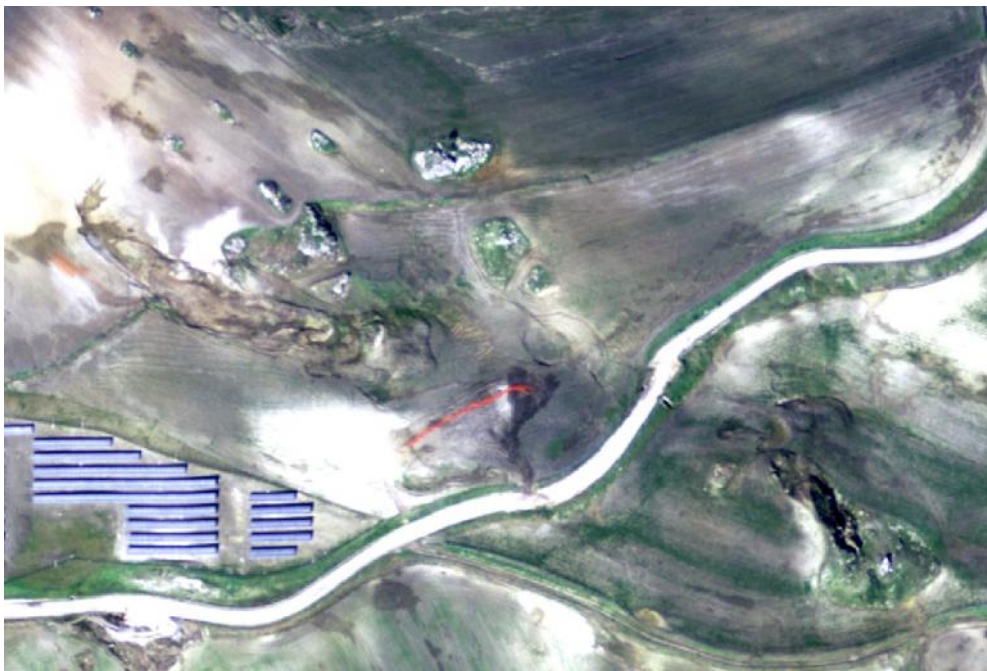
Figure 1 : Orthophoto from March 2011 showing an example of about 100 m wide and few hundred meters long road-damaging landslide that extends from upper left to lower right corner of the image; associated wet areas can be recognized through the tonal differences (darker tones).
